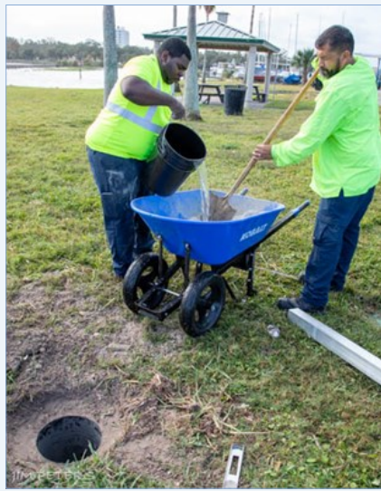
L to R: Dantav Tillman and Edric Diaz mixing the concrete.
