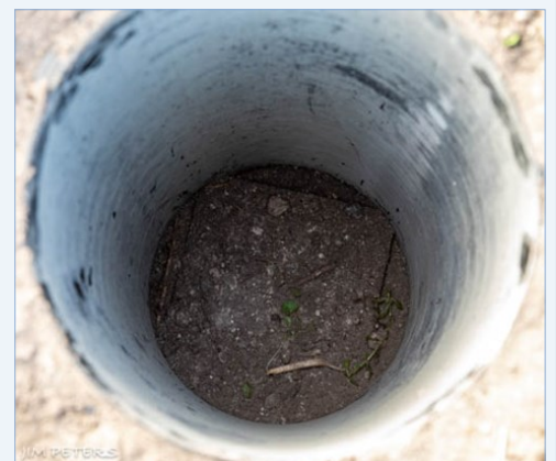
Square stone at bottom of hole to support the ground sleeve.
