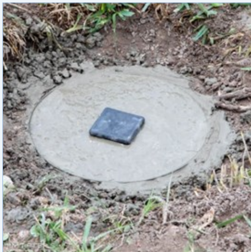
Ground sleeve in concrete with cap to prevent dirt entry. The concrete was very professionally placed around the sleeve. In January the habitat poles will be inserted and the gourds hung to welcome Purple Martins.
