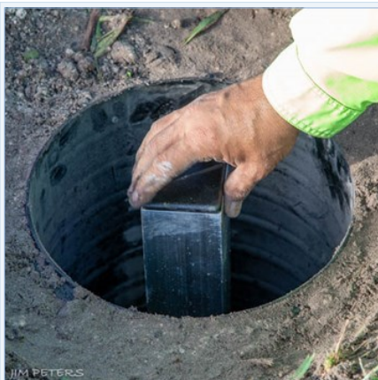
Ground sleeve for later insertion of the habitat pole.
