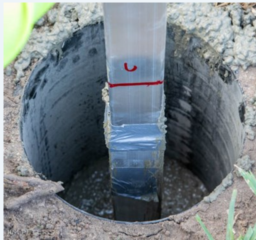
Ground sleeve held in place while concrete is poured.
