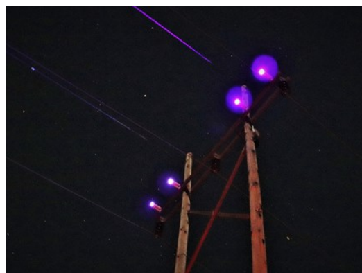
Solar-powered device fitted with ultraviolet lights mounted on transmission lines. Source: media.audubon.org/BirdsAndTransmissionReport.pdf. Photo by James Dwyer
